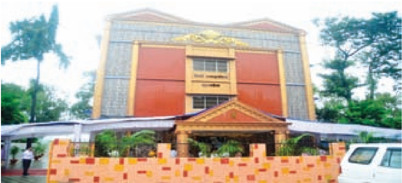
Construction of Resident Dy. Collector/Mamlatdar Office at Khanvel , D&NH with estimated cost of ₹2.60 crore has been completed and inaugurated.
