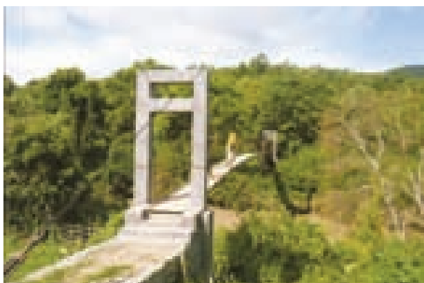
Construction of Suspension Bridge over Tuival river at L. Kanan Village
