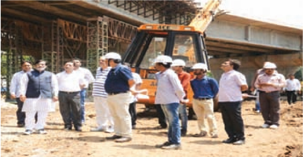
The Hon'ble Administrator of Daman and Diu Shri Praful Patel, is inspecting the construction of Bridge with Senior Officers of the UT Administration of Daman and Diu at Daman.
