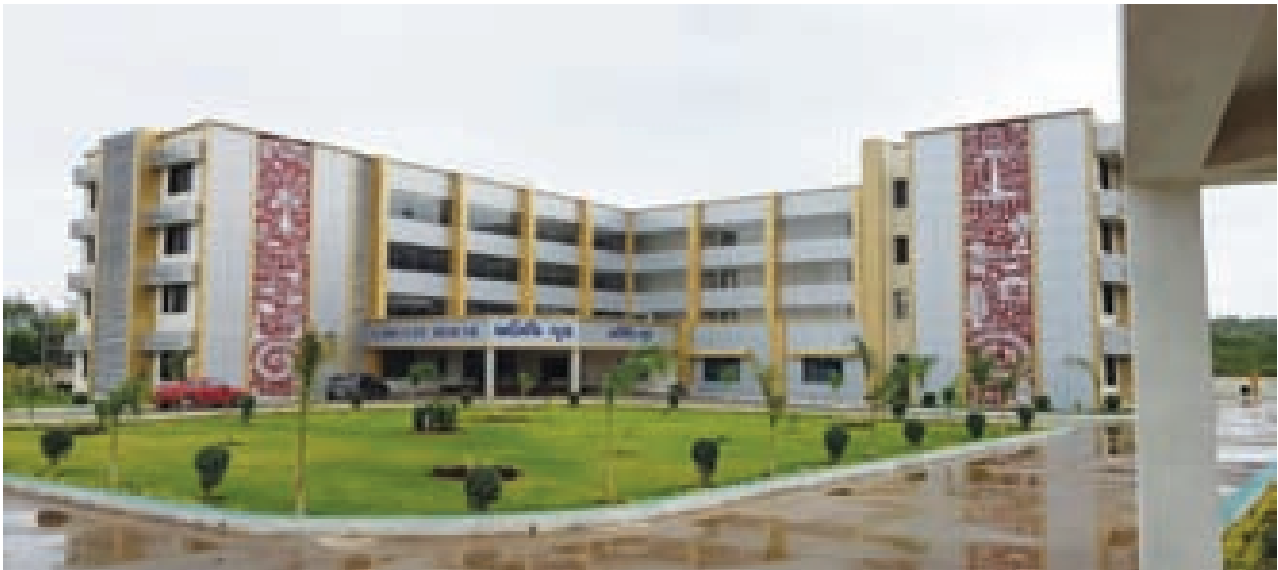
Construction of Circuit house at Silvassa with estimated cost of ₹16.50 crore has been completed.
