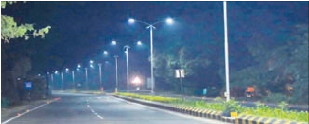
Street lights have been converted into LED lights
