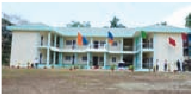
A New Hostel Building of Forest Training Institute at Wimberlygunj
