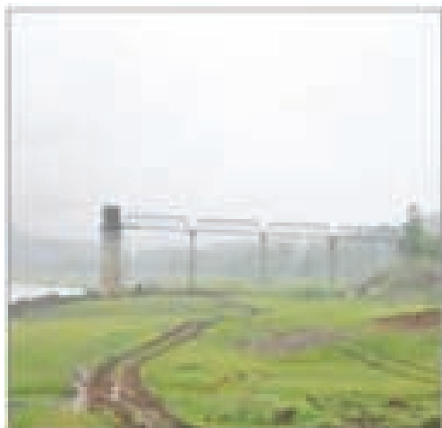
Water Supply Project for Dudhani & Mandoni Patelads
