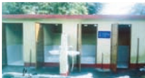
Construction of Public Toilet at Kapra Thaur village (District: Pithoragarh)
