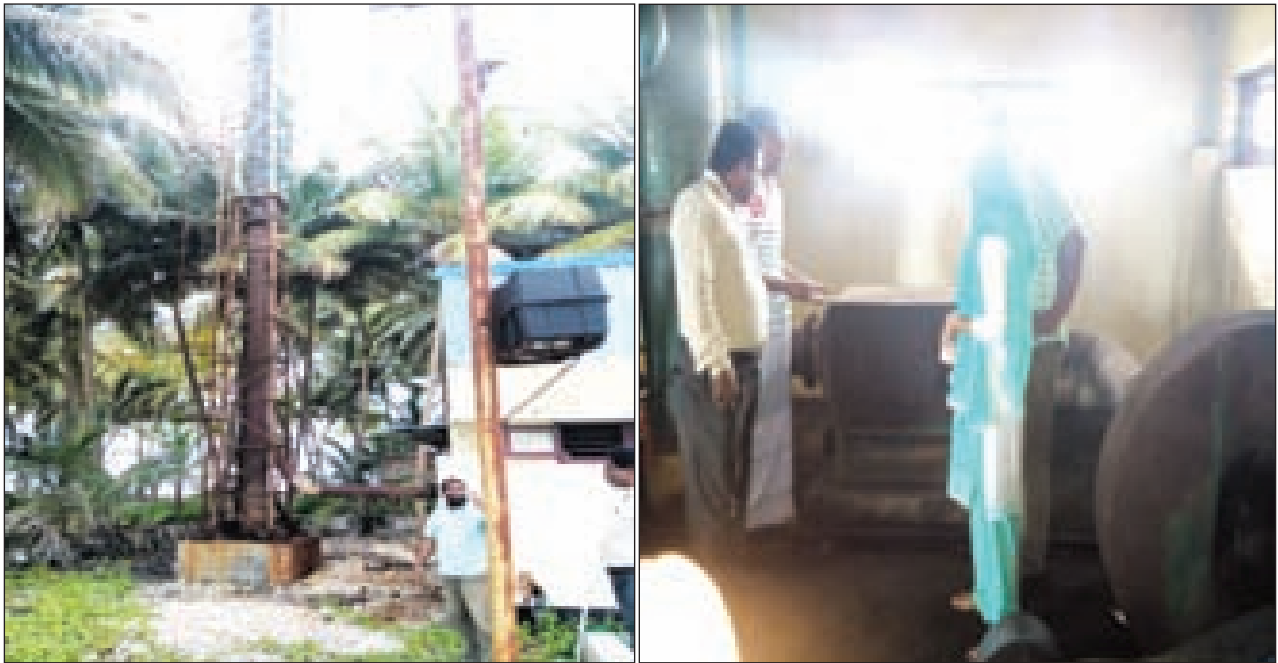
Installation of Incinerators
