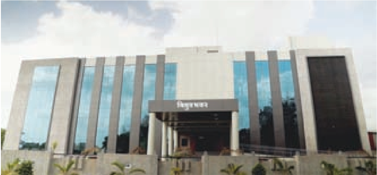
Construction of new office building of Power Department / DNHPDCL With estimated Cost of ₹21.00 crore has been completed and inaugurated.
