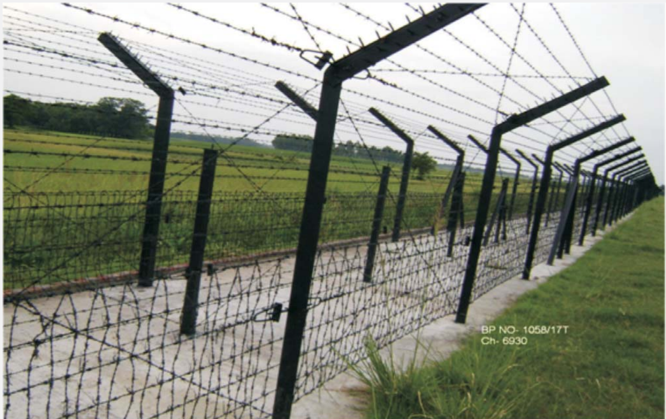
Fencing constructed along Indo-Bangladesh Border
