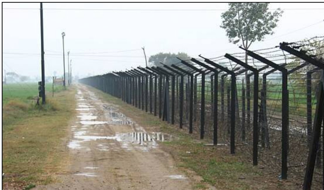
Fencing & floodlighting constructed along Indo-Pakistan border
