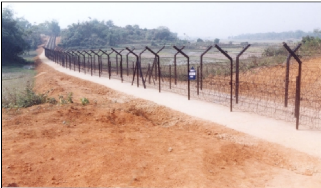
Fencing constructed along Indo-Bangladesh Border
